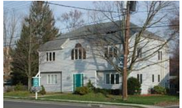
A nice-looking conversion of an apartment building into professional office suites in Madison, CT
