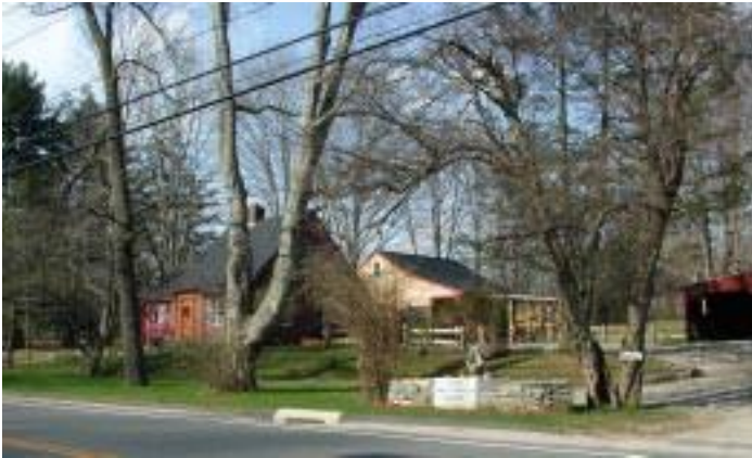
Home with professional office outbuilding, Haddam, CT looks like a traditional New England farm complex.
