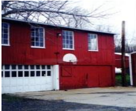
Large, multi-light windows open the appearance of this wall in the Reef Machine works, Middlefield, CT.
