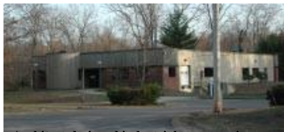
Architect-designed industrial structure in Marlborough, CT with integrated office
