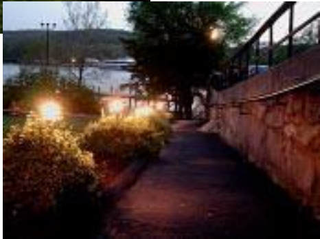
low elevation mounting, shielded pedestrian lighting on walkways,
