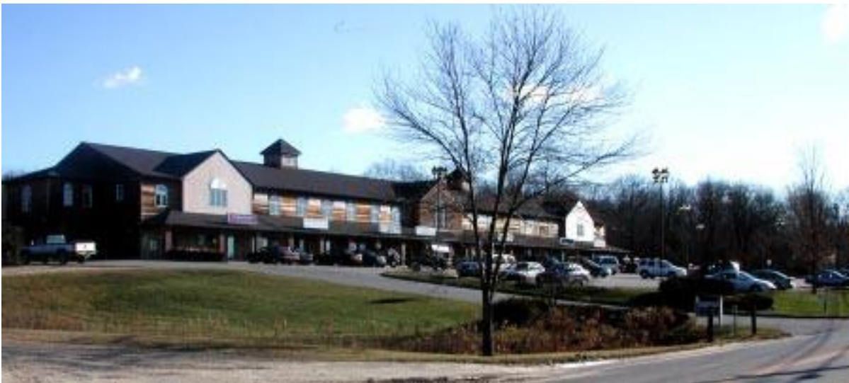
The 12,552 square foot, two-story commercial building at left dominates the Northeast corner at Salem Four Corners, CT.
