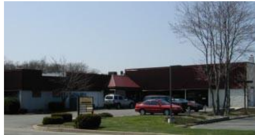
This industrial site in Old Saybrook, CT has no building-related landscaping.
