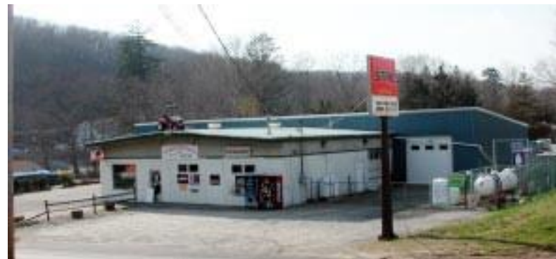
Front view of entry bays and propane tank enclosures on commercial building, Tylerville, CT
